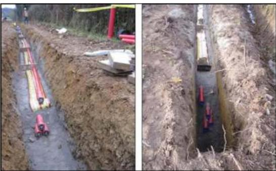
Plate 4-7 Standard Cable Trench View
