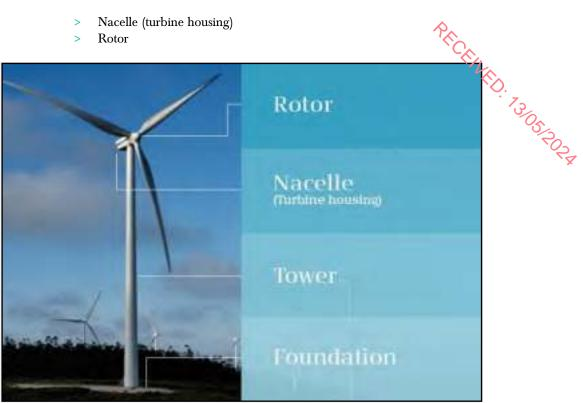
Plate 4-1 Wind turbine components
