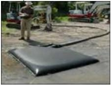
Plate 4-5 Silt bag with water being pumped through
