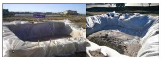
Plate 4-3 Concrete washout area
